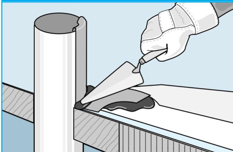
**COMPAFLASH** Flashing tubes are an easy-to-handle solid tube of either APP or SBS modified bitumen compound; the same compound used in our cap and base sheets. The design allows you to heat and trowel additional modified bitumen compound in areas that are difficult to seal. This can be at flashing details, pitch pans and areas of repair.
